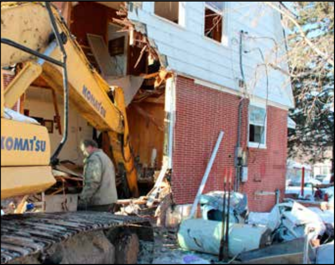
Hengel Ready Mix and Construction plans to begin demolition Jan. 19 or 20. (Staples World photos by Dawn Timbs)
