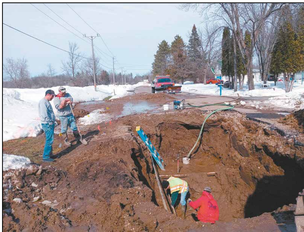
Fixing the water main leak
